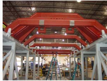
Other Beams used to locate Components in Design Coordinate System Relative to Base Fixture
